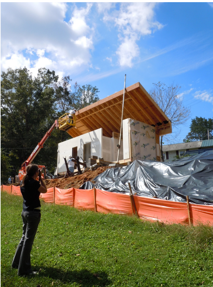
Figure 2. The roof of the first modular unit is hinged into place before temporary supports are installed.
